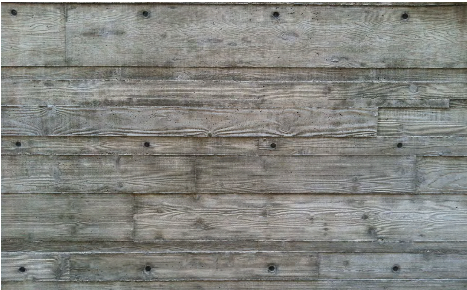
BOARD FORM CONCRETE
